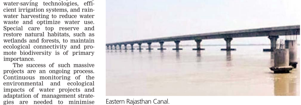
Eastern Rajasthan Canal.
