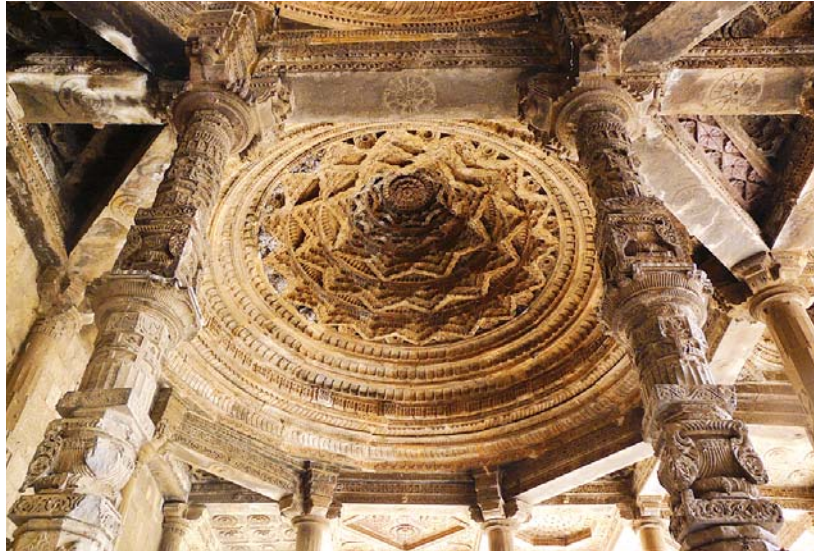
Adhai Din ka Jhonpra Column, beam and dome.
