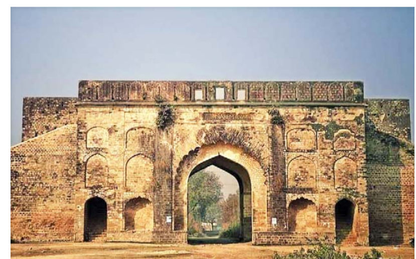
Sultana daku fort.
