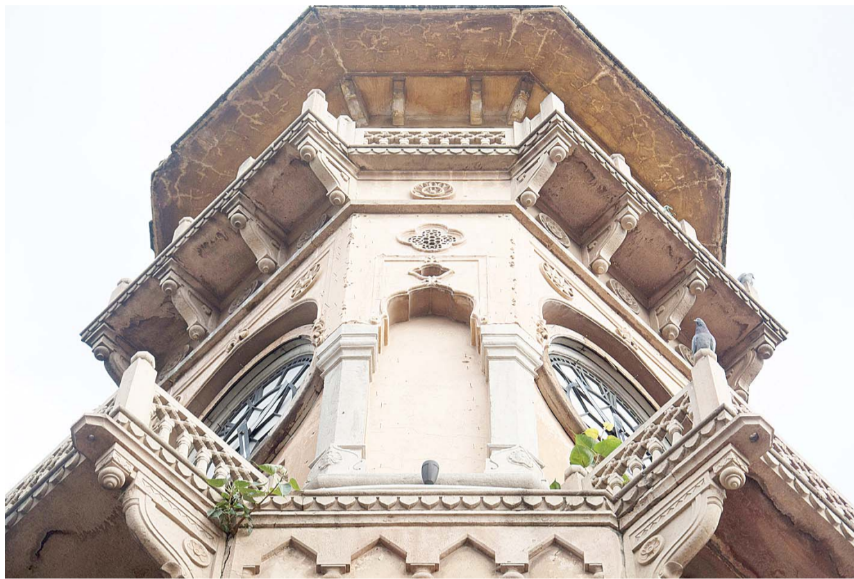
The Yaadgar ghanta ghar with its symmetrical overhanging balconies in rose sandstone and two of the four clock faces visible behind them.
