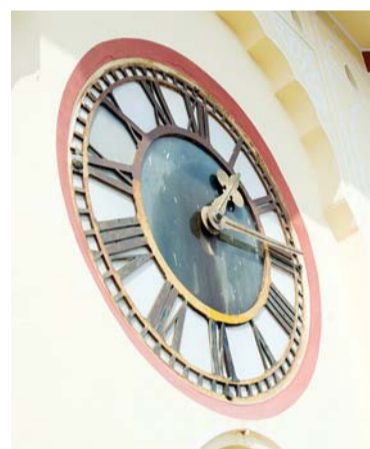
The southern dial of the City Palace Ghanta Ghar. All four clock faces have a circular, painted iron frame at the back of which are attached 25 pieces of glass.
