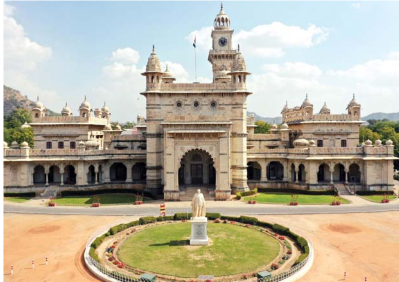
Main building of Mayo College.
