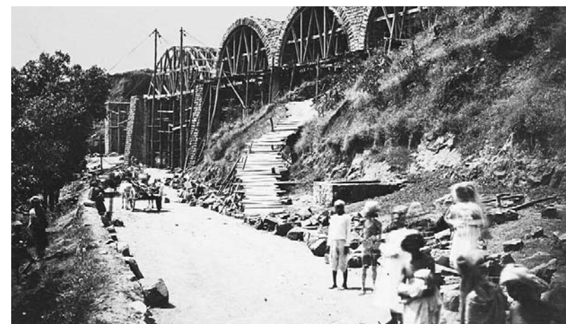
The Reversing-Station Viaduct Ghat Road.
